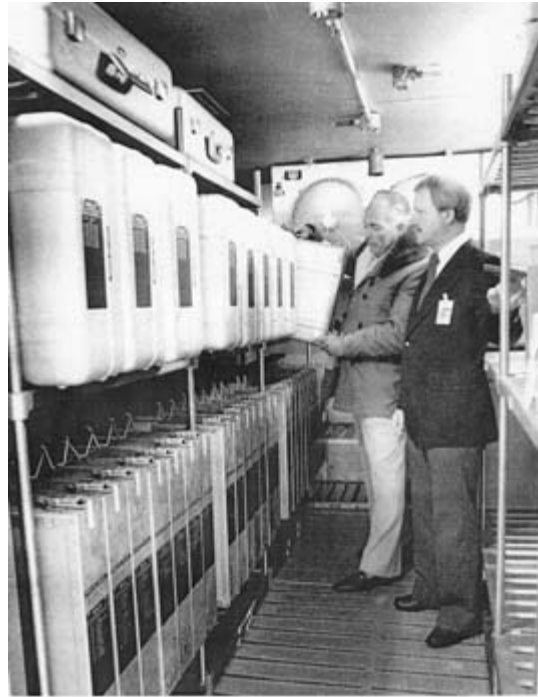
TS_11.jpg - (Photo and caption appeared in Society of Photographic Science and Engineering Journal, October 1987) Frank Zehentner (left) and Terry Slezak prepare to remove an aluminum case containing rolls of original color film from the primary NASA humidity-controlled cold storage vault built for the permanent preservation of spaceflight films. This is one of the two vaults maintained at 0°F (-18°C) and 20% RH located at the NASA facility in Houston, Texas; the other vault, situated in a remote corner of the NASA property, is used to store a complete duplicate set of the films, together with written documentation. A third NASA vault at the White Sands Missile Range in New Mexico, which also operates at 0°F (-18°C) and 20% RH, houses a second duplicate set of backup copies and documentation of the spaceflight films.
